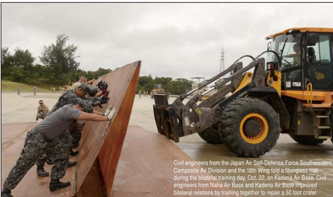
Civil engineers from the Japan Air Self-Defense Force Southwestern Composite Air Division and the 18th Wing fold a fiberglass mat during the bilateral training day, Oct. 22, on Kadena Air Base. Civil engineers from Naha Air Base and Kadena Air Base improved bilateral relations by training together to repair a 50 foot crater.
