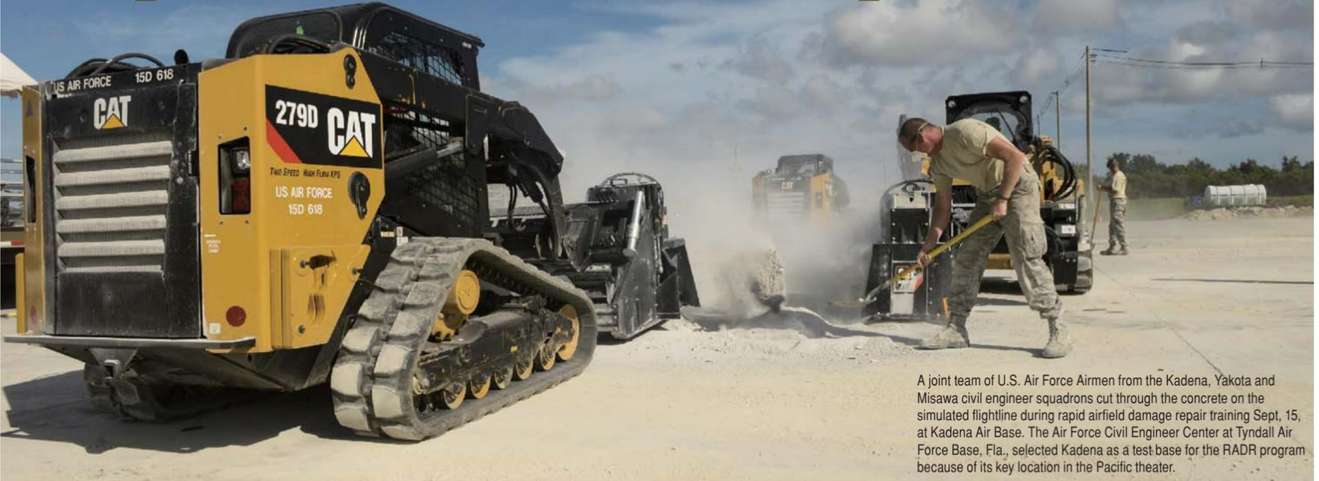
A joint team of U.S. Air Force Airmen from the Kadena, Yakota and Misawa civil engineer squadrons cut through the concrete on the simulated flightline during rapid airfield damage repair training Sept. 15, at Kadena Air Base. The Air Force Civil Engineer Center at Tyndall Air Force Base, Fla., selected Kadena as a test base for the RADR program because of its key location in the Pacific theater.
